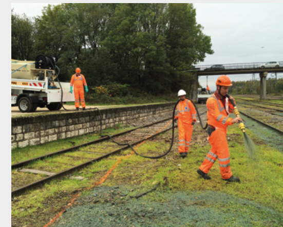
Seeding rail sidings with a hydromulch slurry at Brevans in October 2019 © Anne Petit
